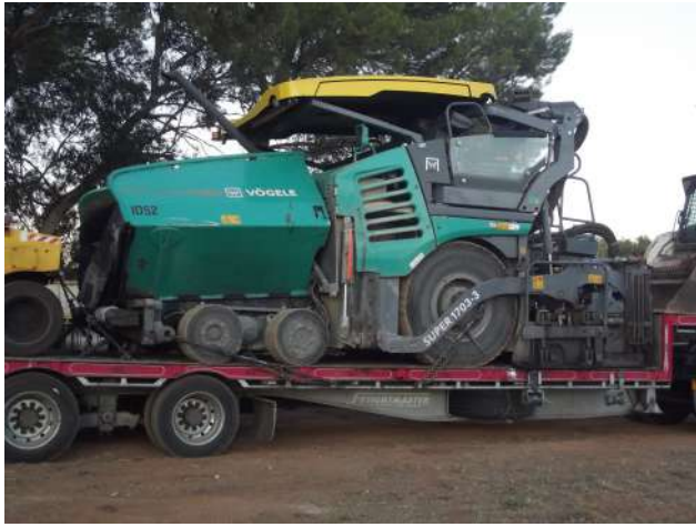
The massive machine used to prepare the surface for painting of the new six court complex at Ewart Oval.
